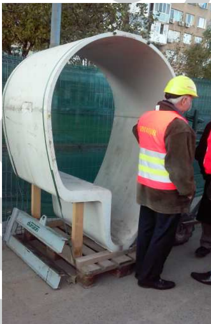
Inlocuire canal colector soseaua Mihai Bravu
